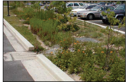
Bioretention Island in Parking Lot
