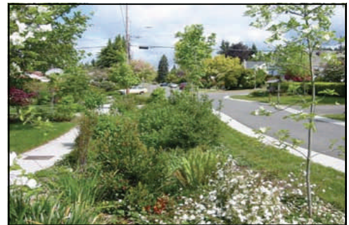
Streetside Bioretention Swale
